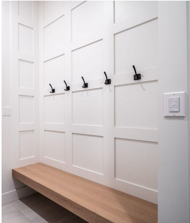
DROP ZONE Trim-built bench with 1x4 wainscoting detail above with 1x4 as cap. Trim detail and cap painted interior trim color. Wood top to be stained white oak.
