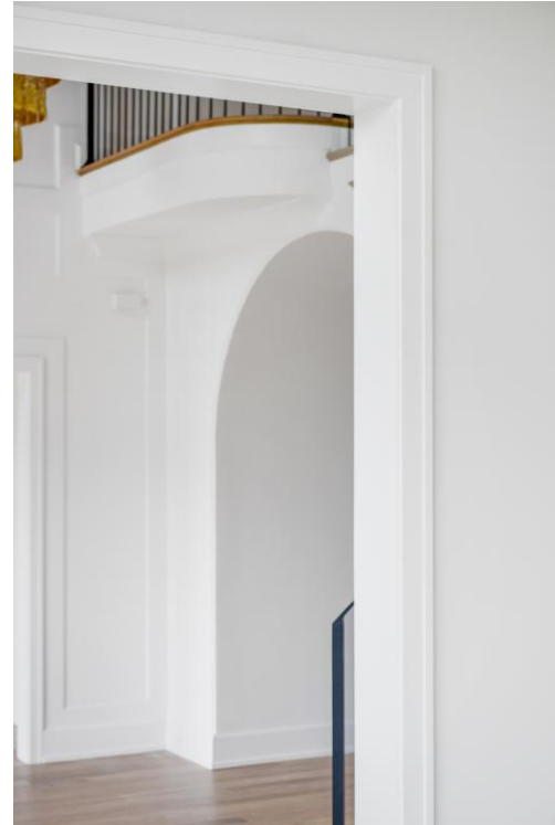
WINDOWS & CASING W-342 Window & door casing throughout. Picture frame windows, no stools.
