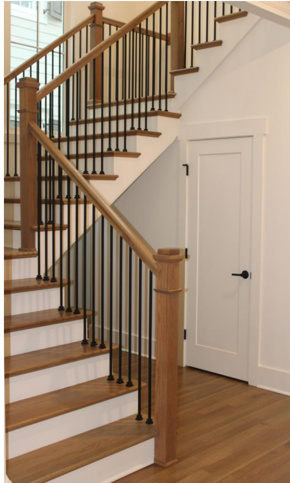
Square iron spindles in black finish Stained square newel posts & standard handrail
